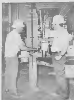
Adjusting the # 5 PS Crude furnace steam demper end observing the draft gauge reading ere Eddy Leclé end R. Benjamin Lampe.
